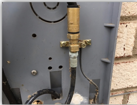
Figure 29: Twist on F-Connector at Ground Block
