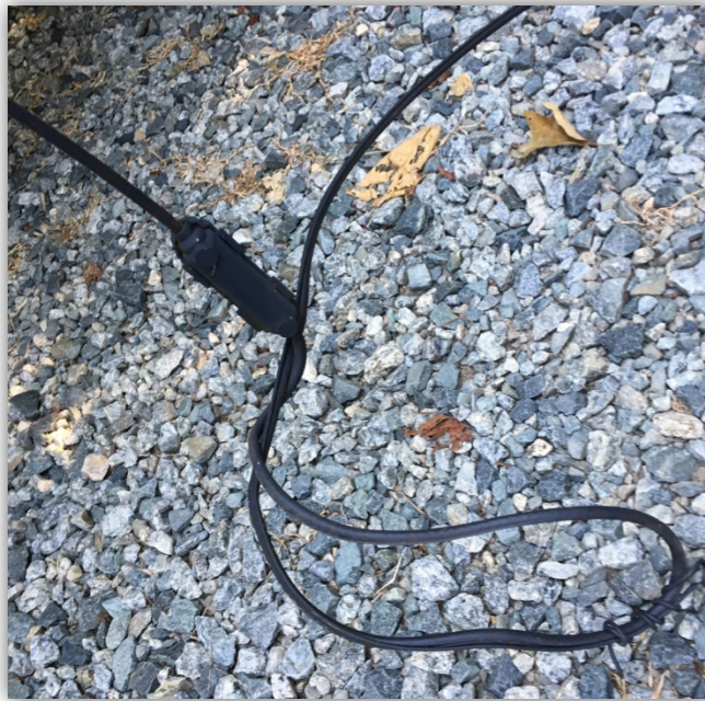
Figure 4: Inline Splice with Weather Enclosure
