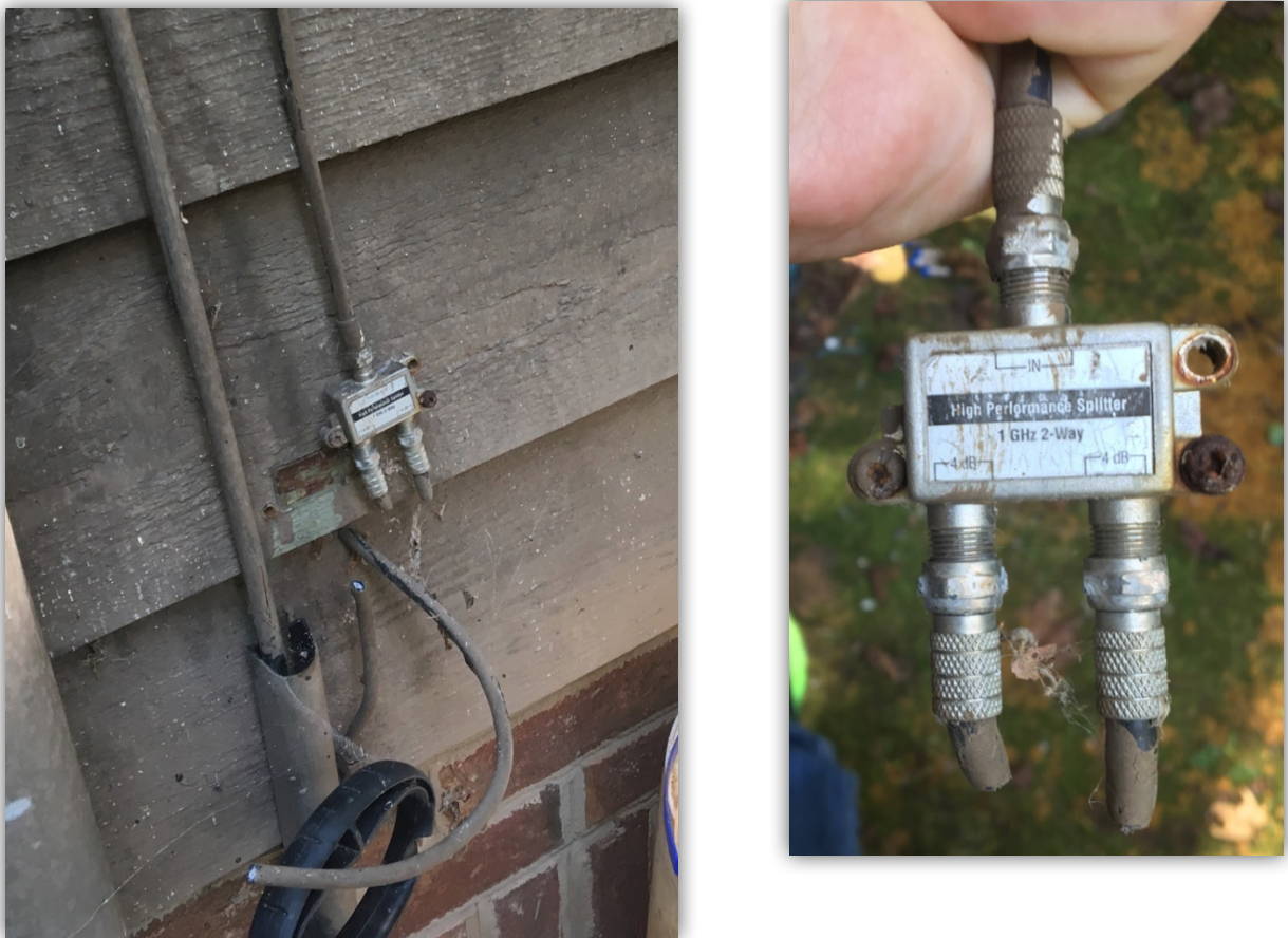
Figure 15: Old Splitter and Push-On F-Connectors
