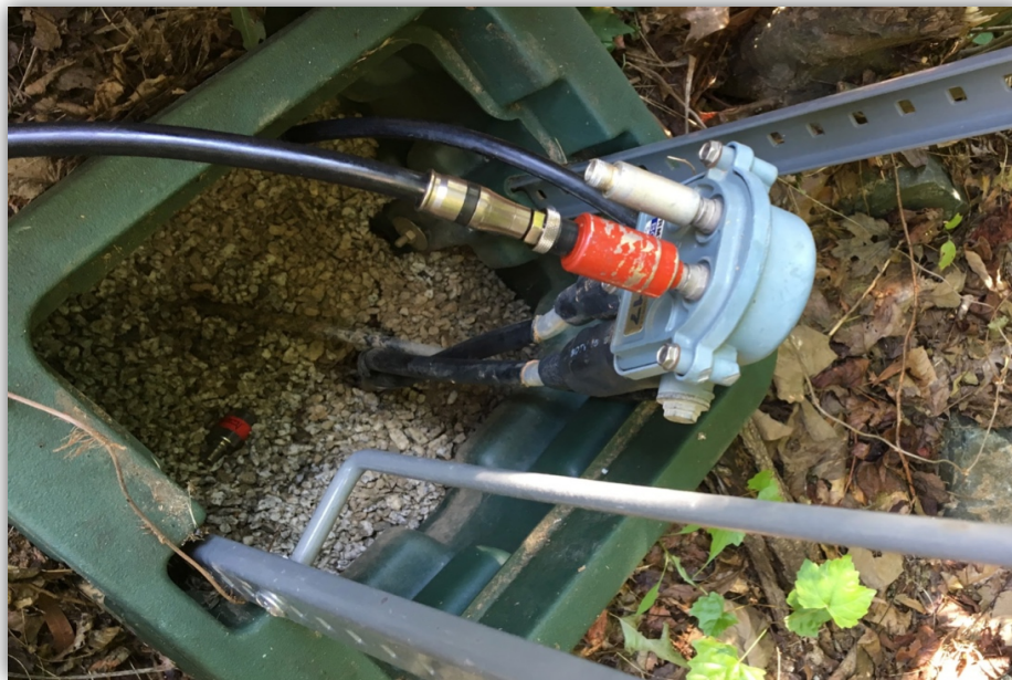
Figure 12: Bad Drop Trap Causing Micro-Reflections
