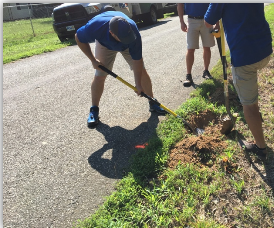
Figure 9: High Leak Location Being Excavated
