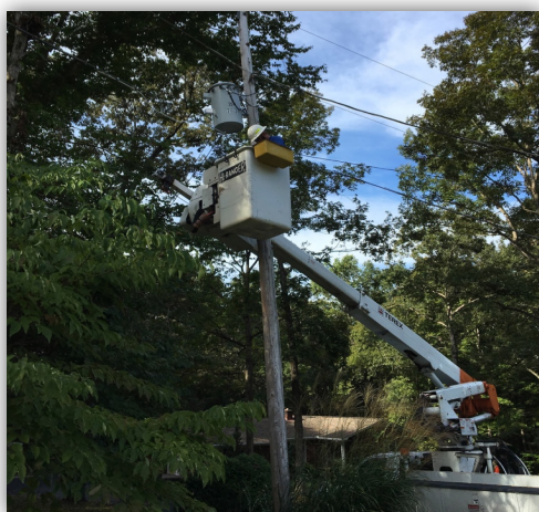
Figure 3: Technician installing M3 Signal Injector
